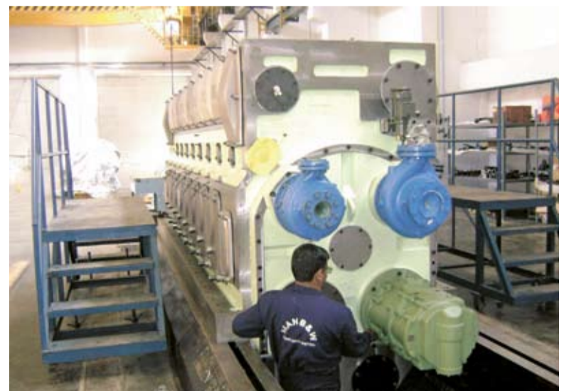
Fitting the lube-oil pump to the new GenSet
