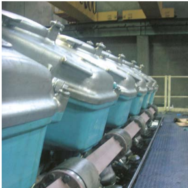
The converted engine's new gas line
